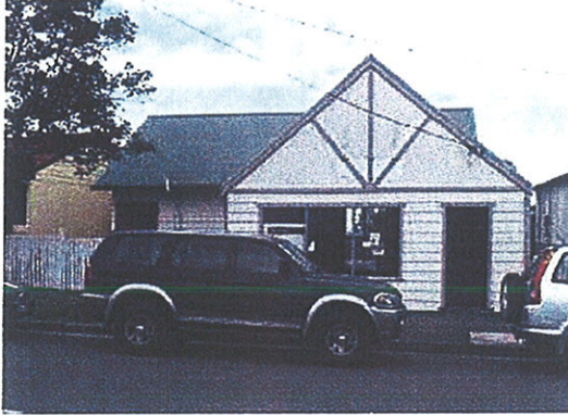
No. 77 Old Bells Line of Road - Vacant
